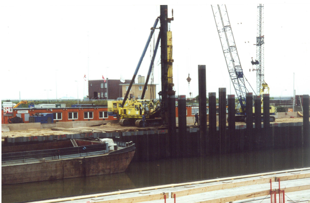
Installation of supporting piles
