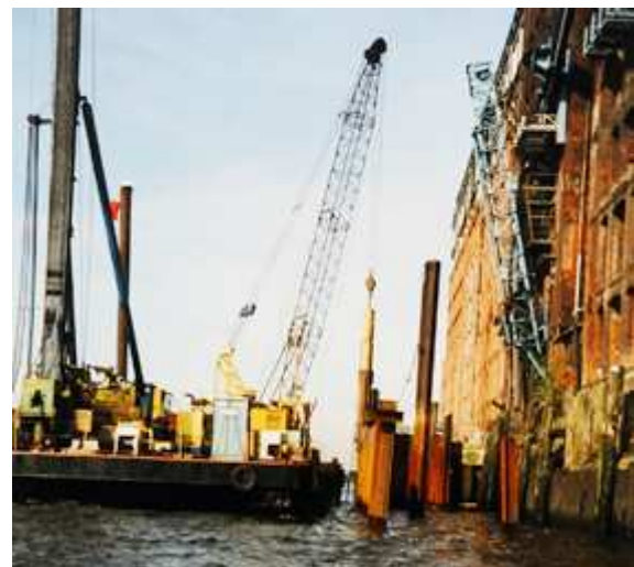
Installation of composite sheet piling on a pontoon
