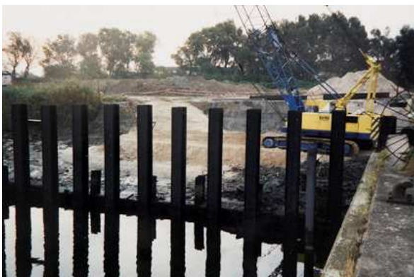
Installed supporting piles
