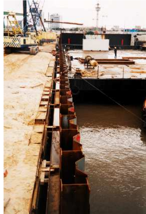
Installed supportin and interim piles
