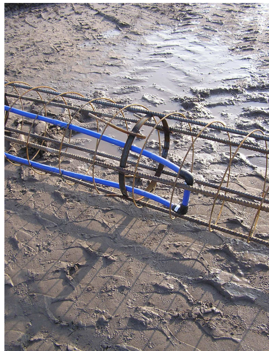
Pipe redirection with electric welding sleeves
