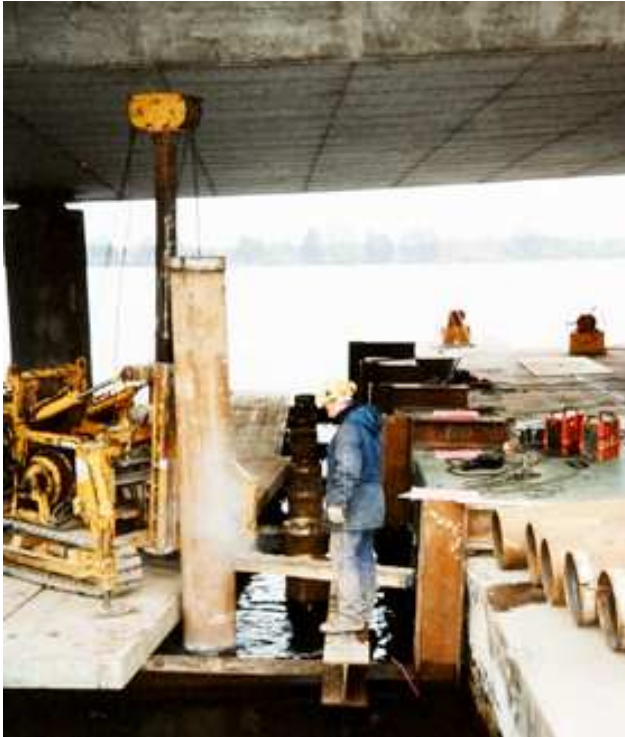
"Mini-Rig" under limited working high - Ø 408 mm
