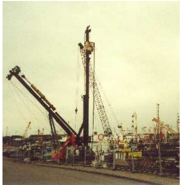
Leader-guided ramming of raked piles
